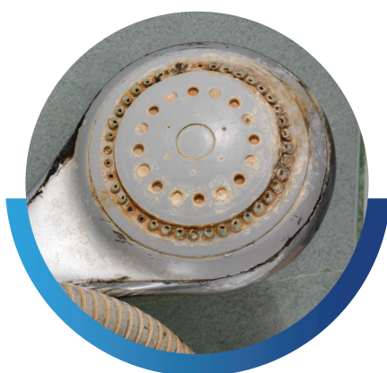
Damage to plumbing systems & reduced flow
